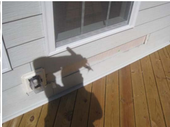
27. [The circle flashing at the water heater exhaust is not installed properly as it will allow water to enter behind the flange.]
