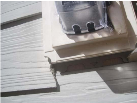
27. [The circle flashing at the water heater exhaust is not installed properly as it will allow water to enter behind the flange.]
