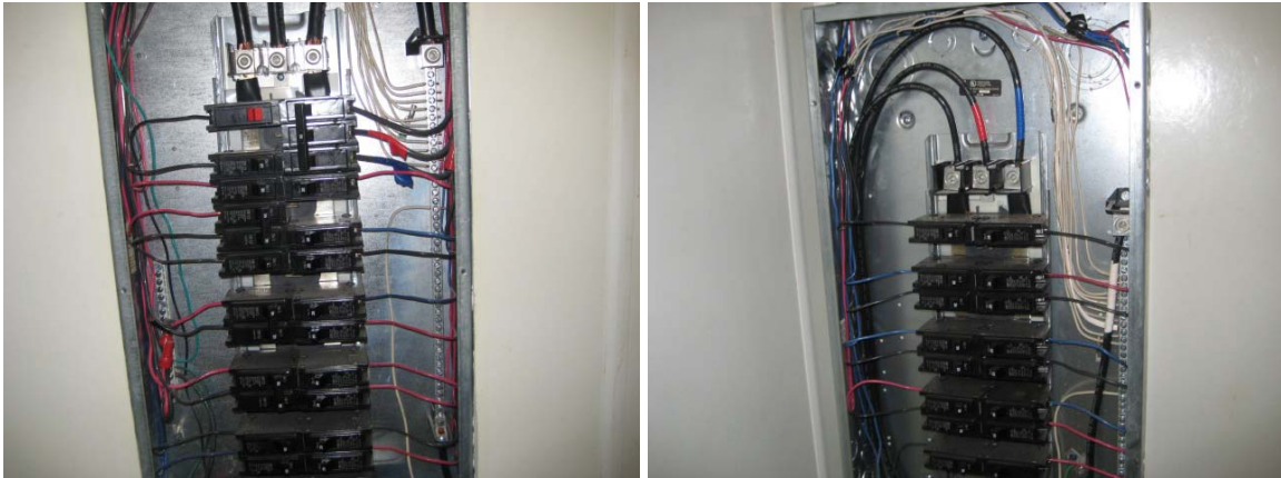
20. [A fluorescent light in the office ceiling does not turn on.]
